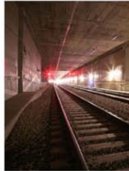
CRITICAL ZONES SUCH AS AN EXISTING TUNNEL, BRIDGE OR UNDERPASS WHERE A REDUCTION OF THE BALLAST THICKNESS IS NEEDED
